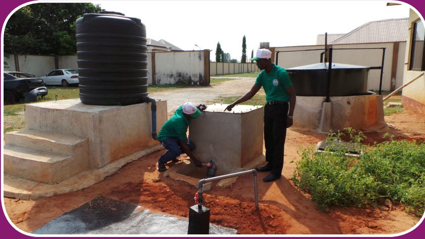
Mr. Peter Ibrahim (left) and Mr. Ifeanyi Aghaulor adjust the waste outlet pipe of the household biogas digester at the Government Guest-house Kitchen, Asaba, Delta State, Nigeria.
